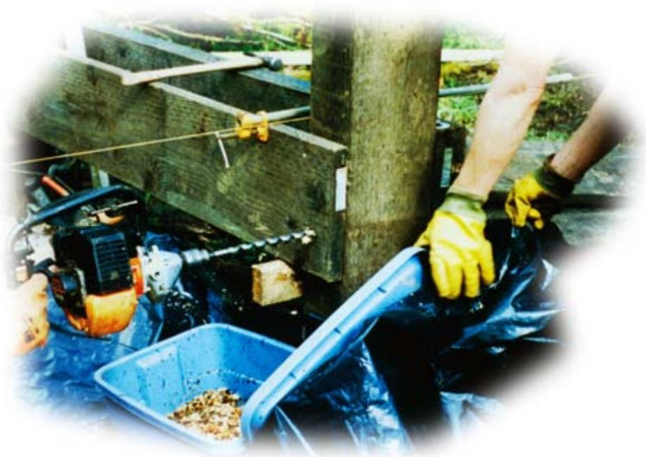
Figure 9—A tub can be used to collect sawdust when drilling preservative-treated wood. Collecting debris during construction helps to minimize environmental impacts.
